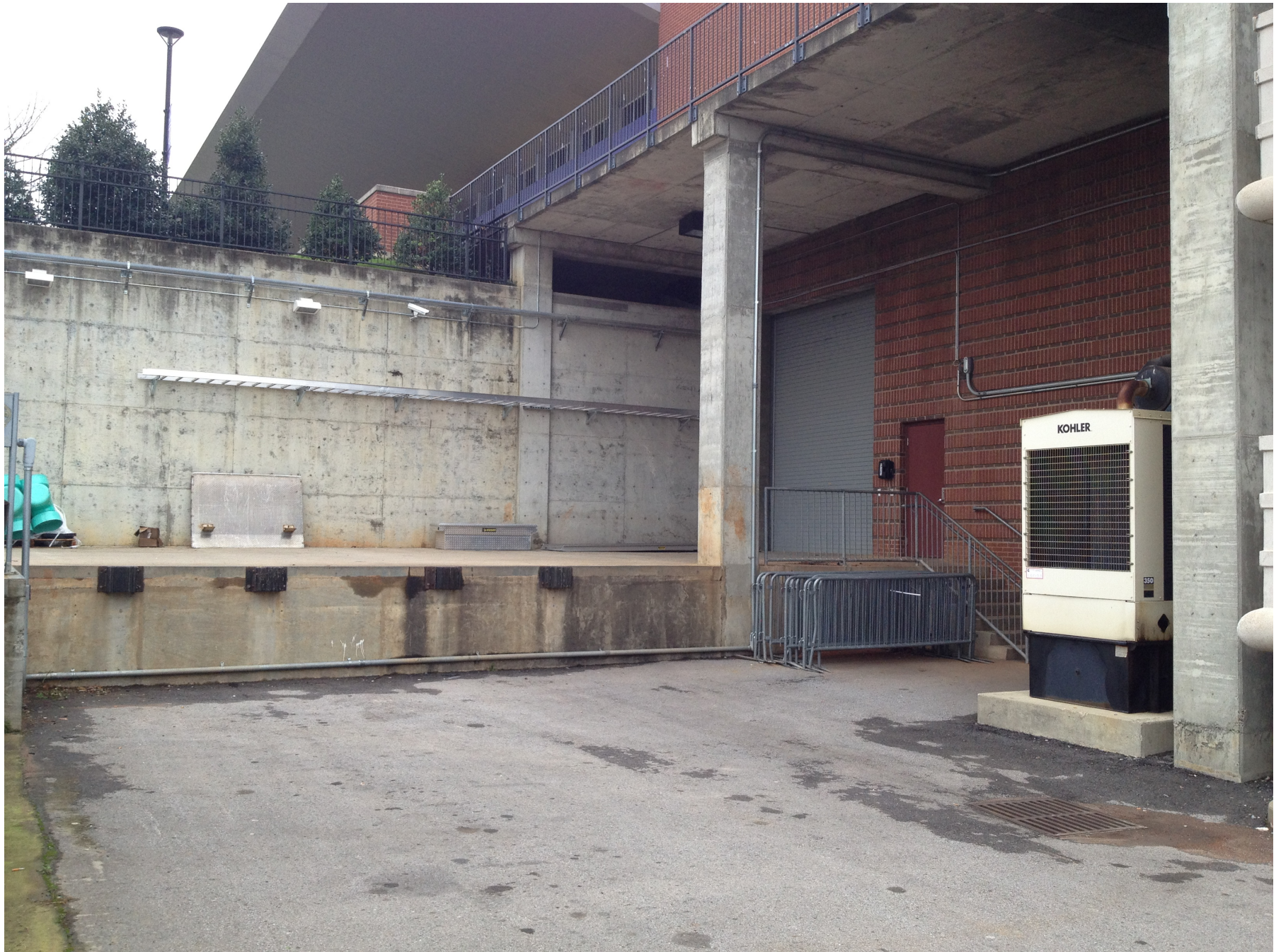
View of loading dock and door.
